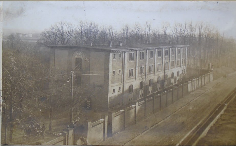
View of "A" Building.
